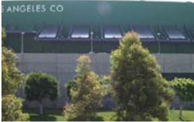
LACC South Hall 150 kW Solar Canopy
